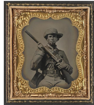
Pvt. Alldredge, Co. A, 48th Alabama
